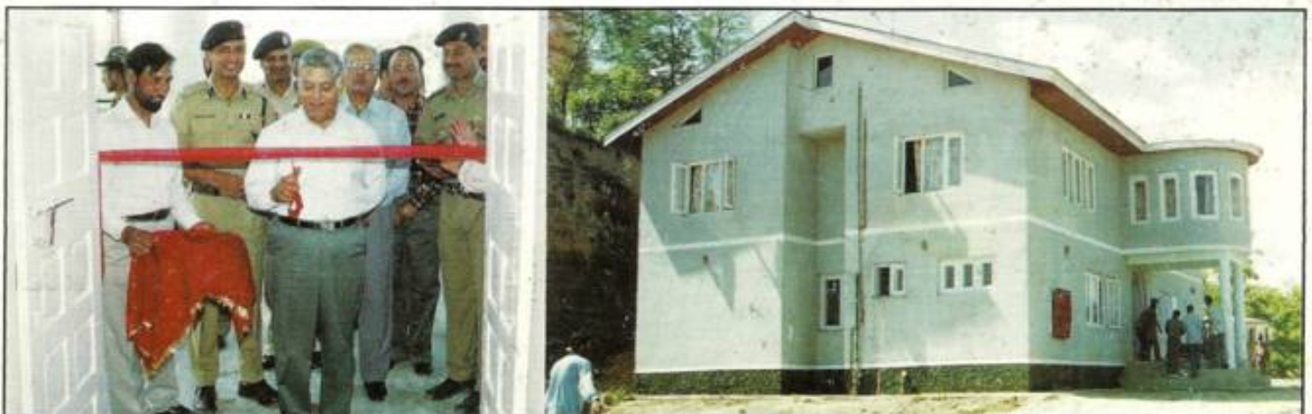
Shri A.K. Suri, the then DGP, J&K inaugurating the newly constructed building of Police Division Humhama (Budgam) on May 18
